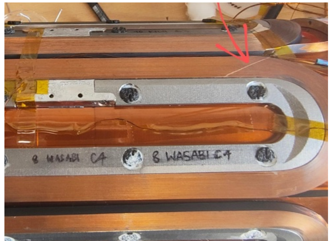
Fig. 18: Physical damage observed in Coil 4 HTS tape attributed to tool contact during manufacturing, correlating with the electrical performance degradation observed during testing.
